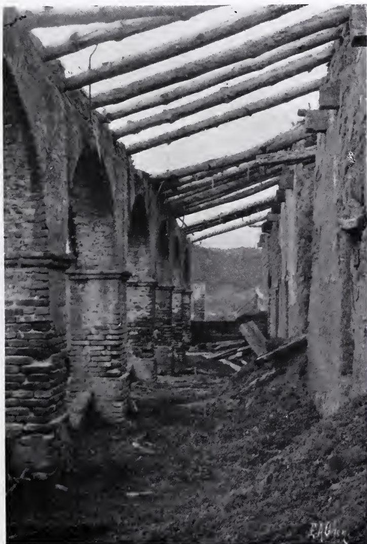
ONCE CLOISTERS: NOW CRUMBLING RUINS.
